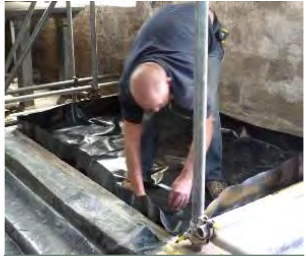
Damp proof membrane being fitted in the base of the monument.
